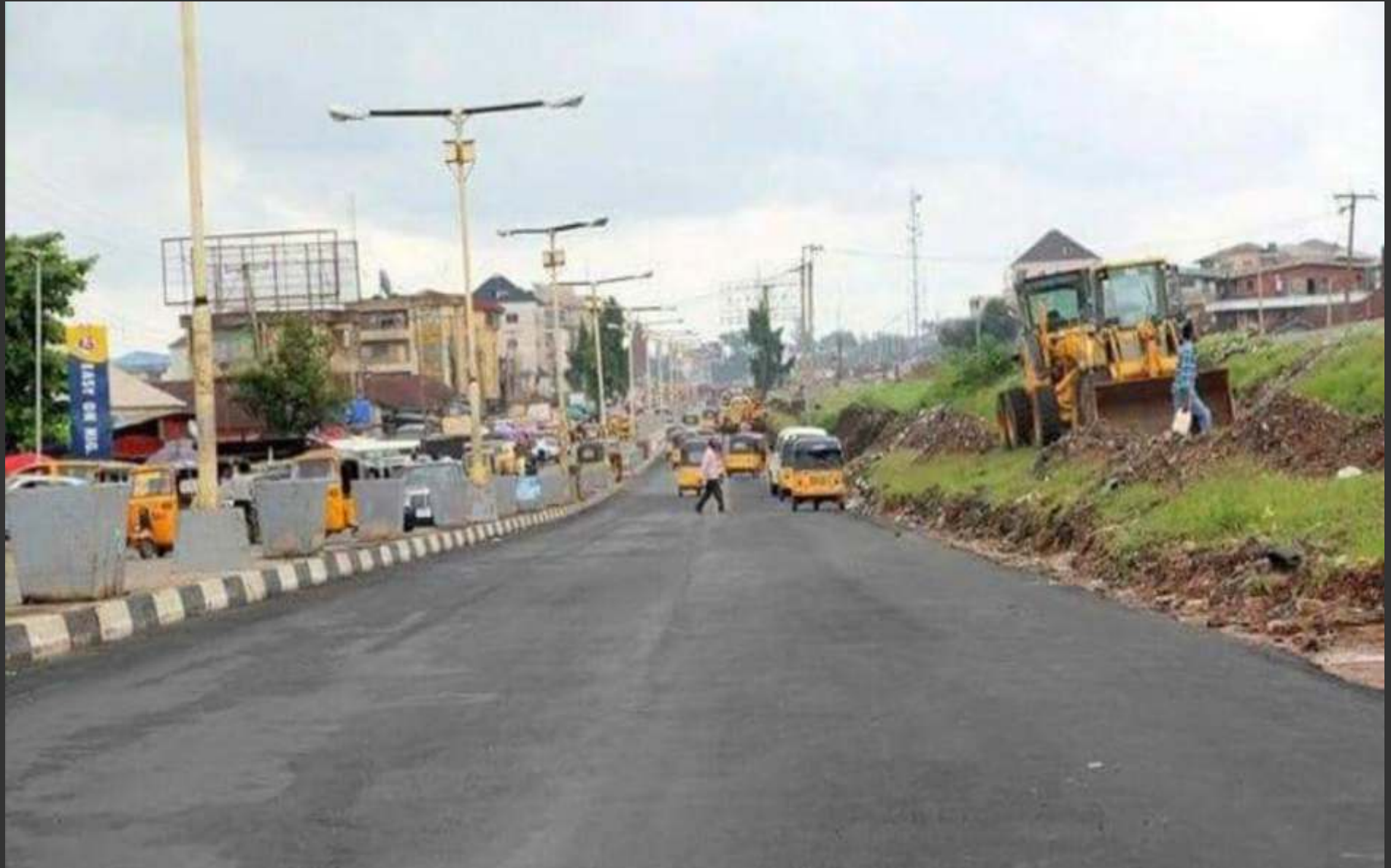
RE-ASPHALTED UMUWAYA ROAD UMUAHIA
