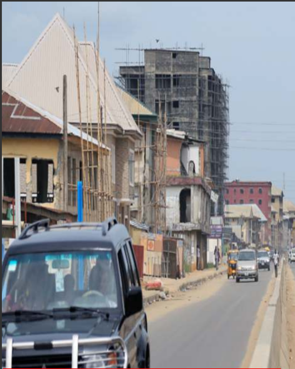
NEW FAULKS ROAD, ABA (SEVEN DECK AXIS AFTER)
