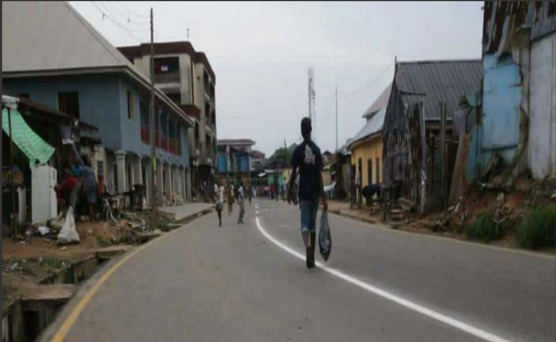
CONSTRUCTION OF IBADAN ROAD, ABA
