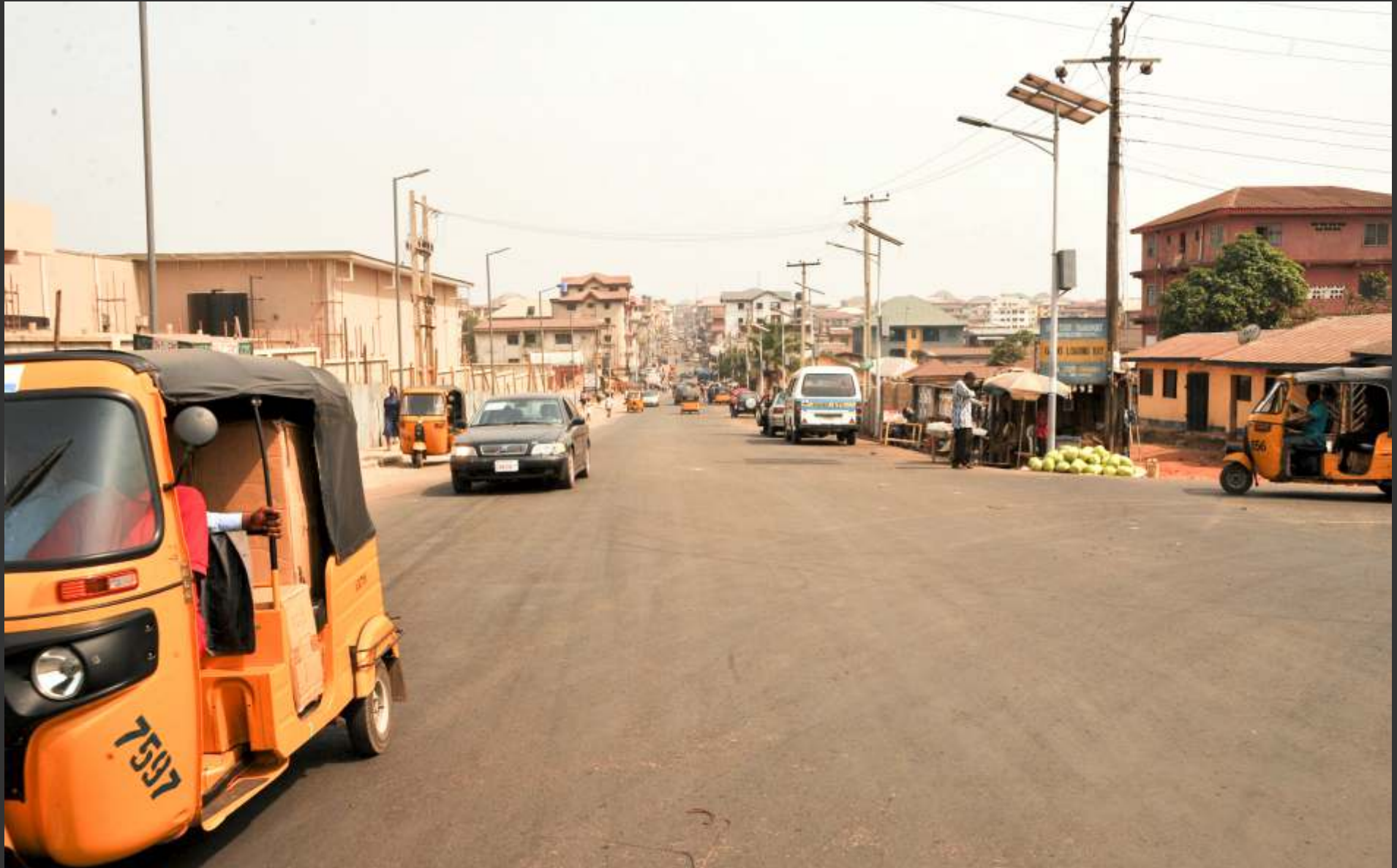
RE-ASPHALTED UWALAKA STREET UMUAHIA
