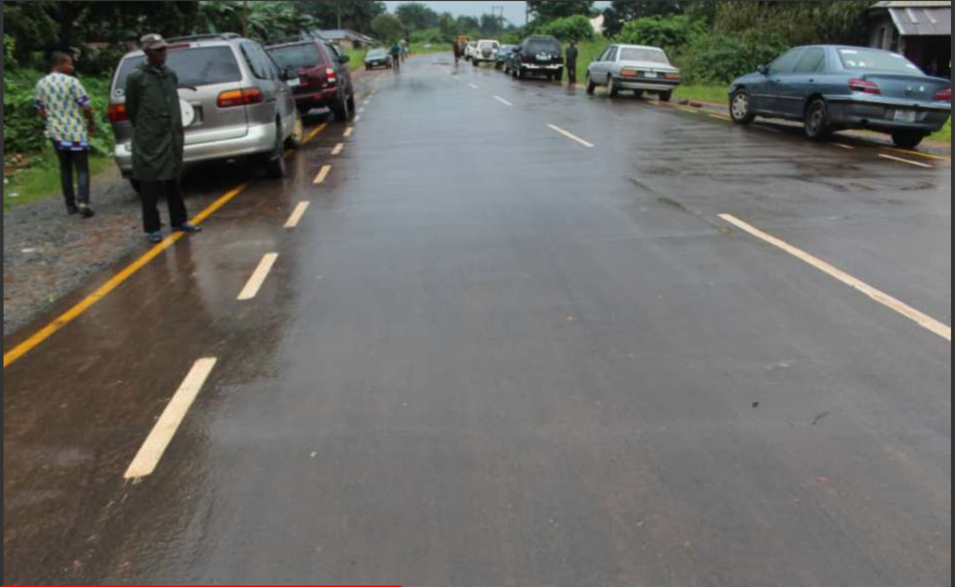
OMOBA-UMUENE ROAD, ISIALA NGWA SOUTH LGA
